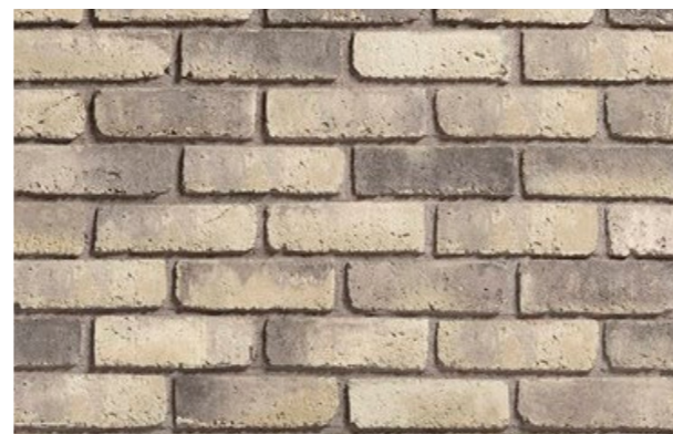
Heritage buff brick to elevations to street
