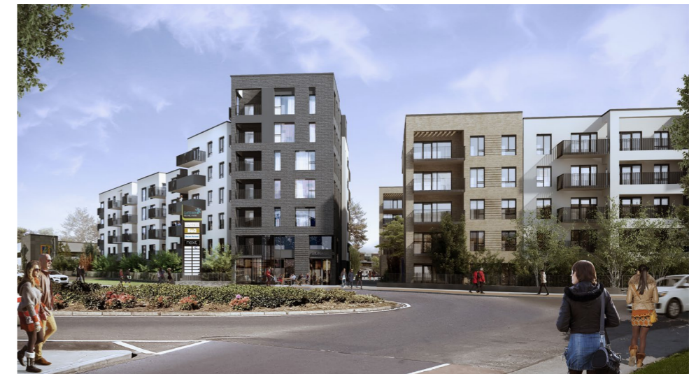
View to front of Block B at corner of site on Western Bypass
