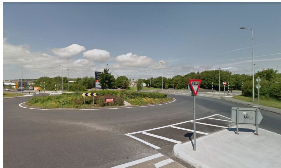
View of entrance to site from Western Distributor road
