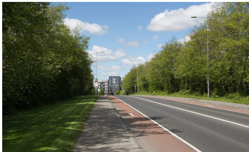
View along Western Distributor Road towards Block B, from the City approach
