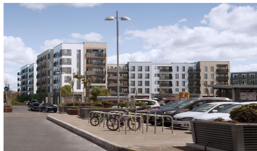
View of Block D from the existing carpark
