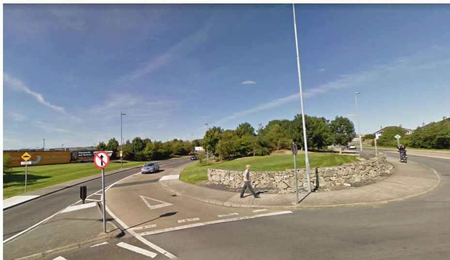
Roundabout entrance to site
