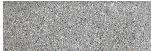
Reconstituted stone cladding to lower levels
